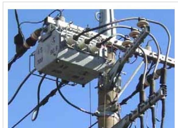
Fig. 1 A Pole Mounted Switch
